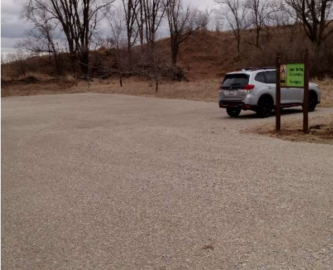
New parking lot put in over the winter with additional trail signage.
