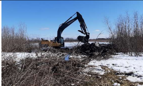
East Pond Berm Under Construction
