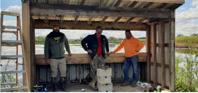
Cody, Steve & Rich – Installing Blind #2
